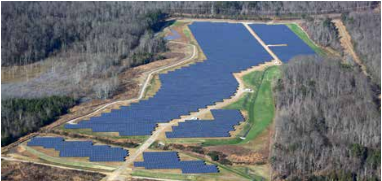
The Volkswagen Chattanooga Solar Park has a peak output of 9.5 megawatts and is the largest solar facility operated by any carmaker in the USA. This eco-friendly power will be used in production of the Passat.
