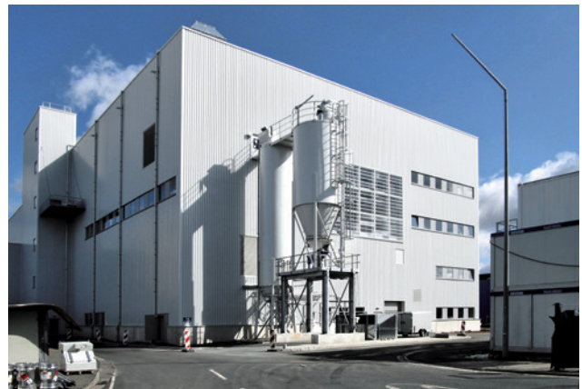
The new plastics paintshop in Wolfsburg.
